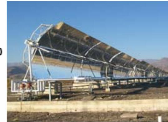
"Parabolic trough collectors producing directly superheated steam (Courtesy of DISS - 2)"
